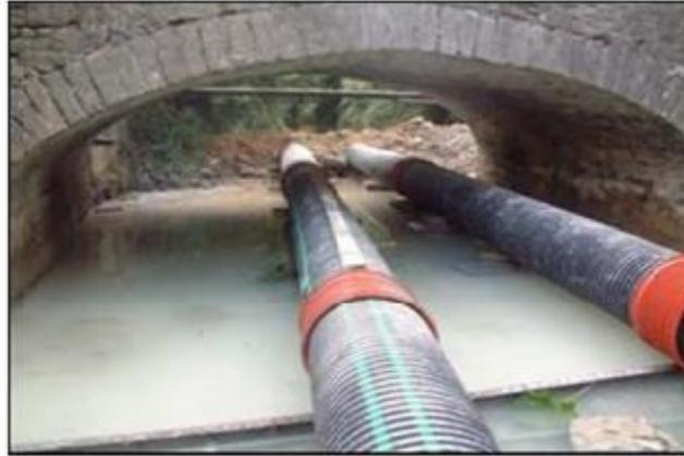
**Plate 2.** Passive diversion of stream through dry works area.
